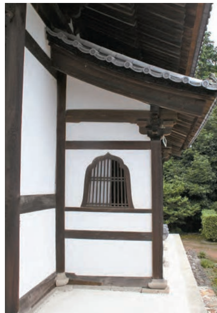
Figure 10. Photograph of extension to Dharma hall.
