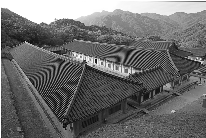
FIG. 1.4. The Canon Storage Hall (Changgyönggak). Courtesy of Haein Temple, Mt. Kaya National Park, South Kyöngsang Province, South Korea.
