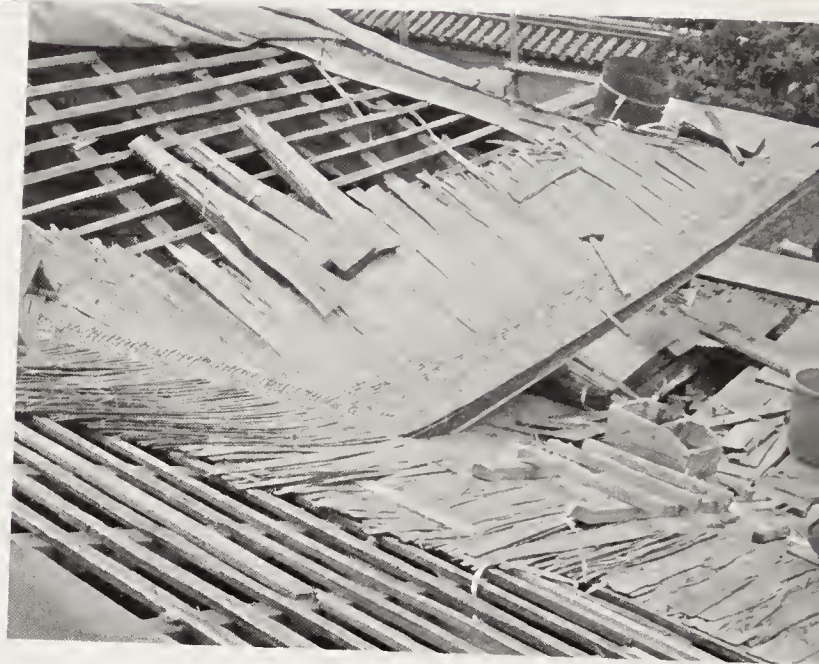
91. Narrow, yard-long strips of cedar bark are put on in layers.
