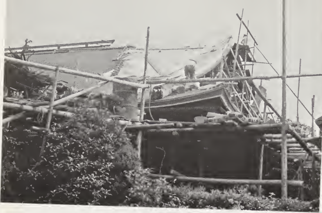
90. The cedar bark roofs of the temples need to be replaced every thirty years. The old roof is removed in sections and the exposed area is covered with a tarpaulin during the night in case of rain.
