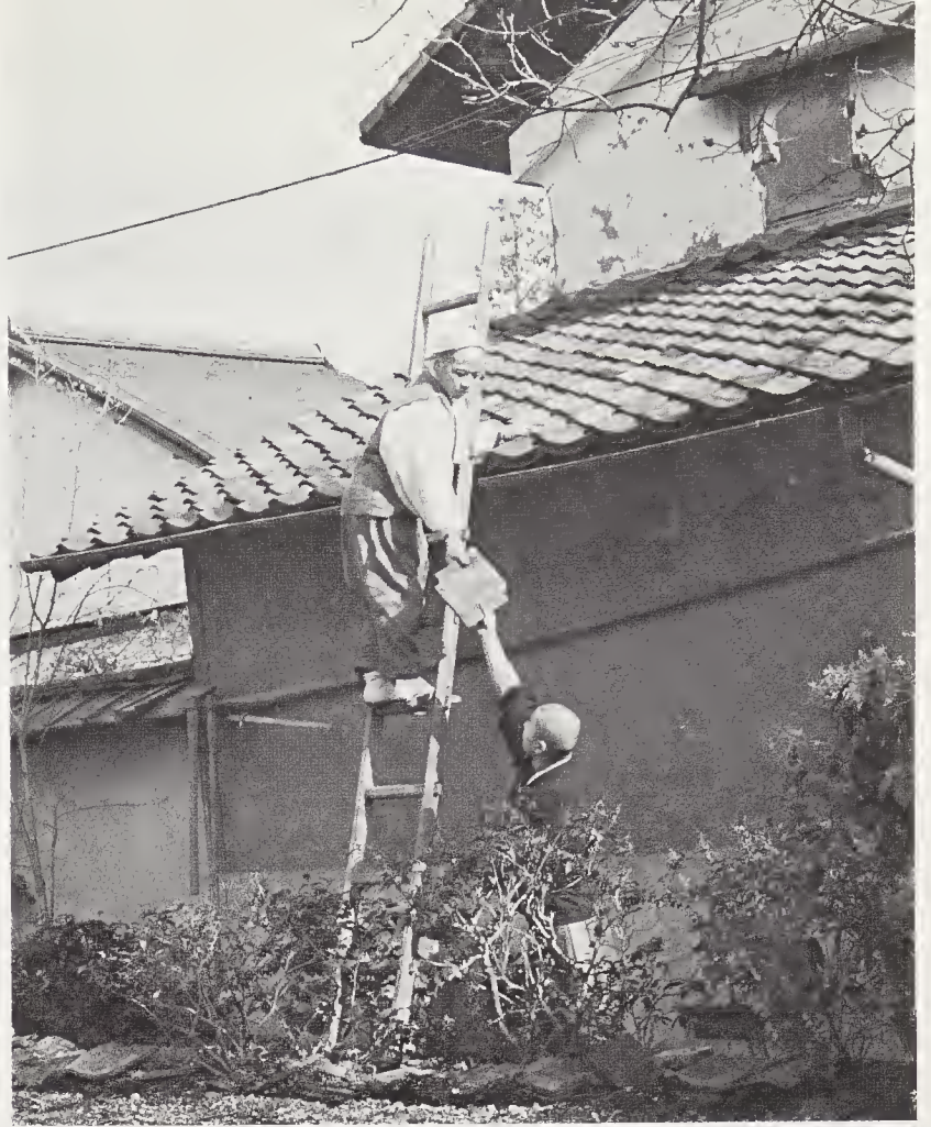
83. 4:30 P.M. Minor repairs are carried out in any spare moments.
