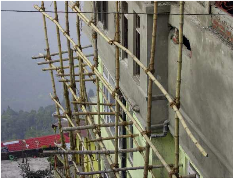
Bamboo is the material of choice for construction scaffolding throughout Asia, as here in Gangtok, Sikkim.
