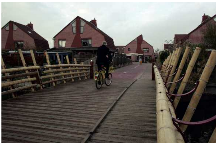
A modern-day bridge built of bamboo in the Netherlands, designed by Pim de Blaey and Charley Younge.
