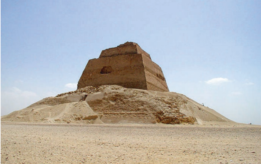
Fig. 3.5 The pyramid at Meidum, in Egypt, as it appears today. It was to be the largest pyramid ever built at its times but it collapsed during construction. Image from Jon Bodsworth – http://www.egyptarchive.co.uk/html/meidum_02.html
