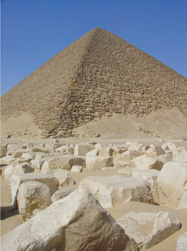
Fig. 3.7 The “Red Pyramid in Dashur. A large building, but much less impressive than the well-known pyramids of Giza. It was built at a low angle probably because the architects feared a collapse like the one that destroyed the Meidum pyramid. Image by Ivrienen at English Wikipedia , creative commons license
