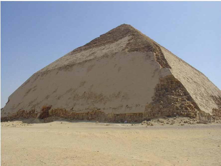
Fig. 3.6 The “bent” pyramid at Dahshur, Egypt. The curious shape of this building was probably the result of the attempt to avoid it suffering the same fate as that of the collapsed pyramid at Meidum. Image by Ivrienen at English Wikipedia , creative commons license
