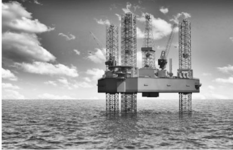
FIGURE 1.6. The Deepwater Horizon, the offshore oil rig at the epicenter of the BP disaster, was harvesting ultra-deep oil, one of the nonconventional resources increasingly exploited by the fossil-fuel industry.
