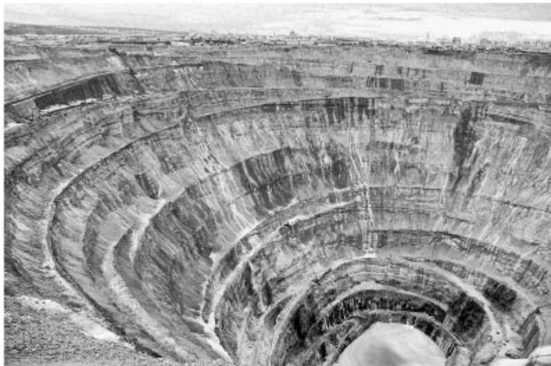
FIGURE 6.2. The remnants of the diamond mine of Mir, in Yakutia, eastern Siberia, Russia. Diamonds are mined in open pits and require vast excavations to recover relatively small amounts. The now-inactive Mir mine is so deep that the atmosphere above it has changed, and the surrounding airspace was closed to helicopter traffic after several were pulled downward by the airflow.
