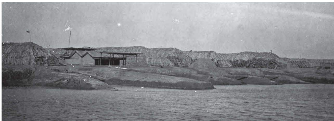
Fig. 11 Photographs of the giant salt heaps along the Hai River, southern section of the Austro-Hungarian concession around 1902, today stored in the Austrian War Archives, Photographic Collection, and published in Winterhalder’s Kämpfe in China (1902, 39) [Austrian State Archives, Department of Kriegsarchiv ]
