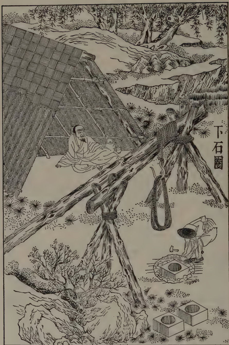
Figure 5-7. Lining a drilled shaft with stones [Ch'ing addition].
