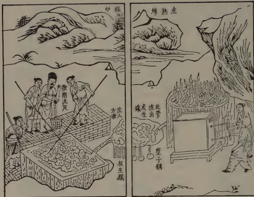
Figure 14-10. Smelting iron ore to make pig iron and wrought iron. Blast furnace at right and puddling pit at left.
