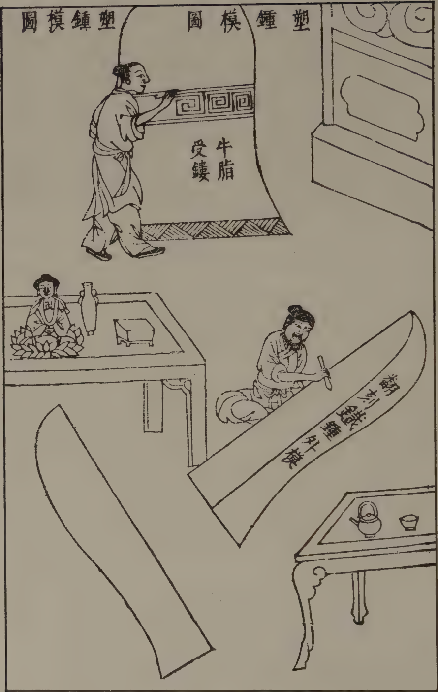
Figure 8-1. Mold for bell.
