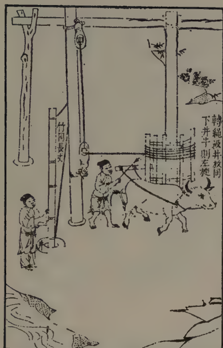
Figure 5-8. Drilling a salt well in Szechuan.
