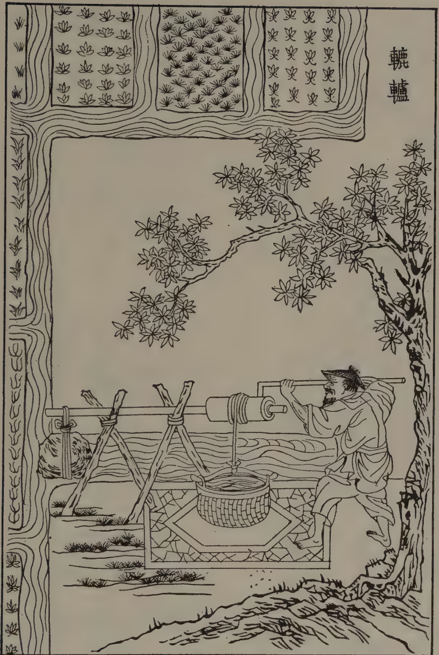
Figure 1-14. A pulley wheel [Ch'ing addition].
