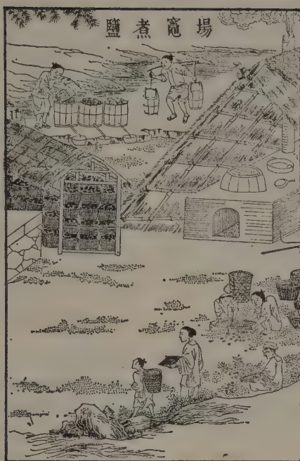
Figure 5-12. Boiling and crystallizing salt brine [Ch'ing addition].
