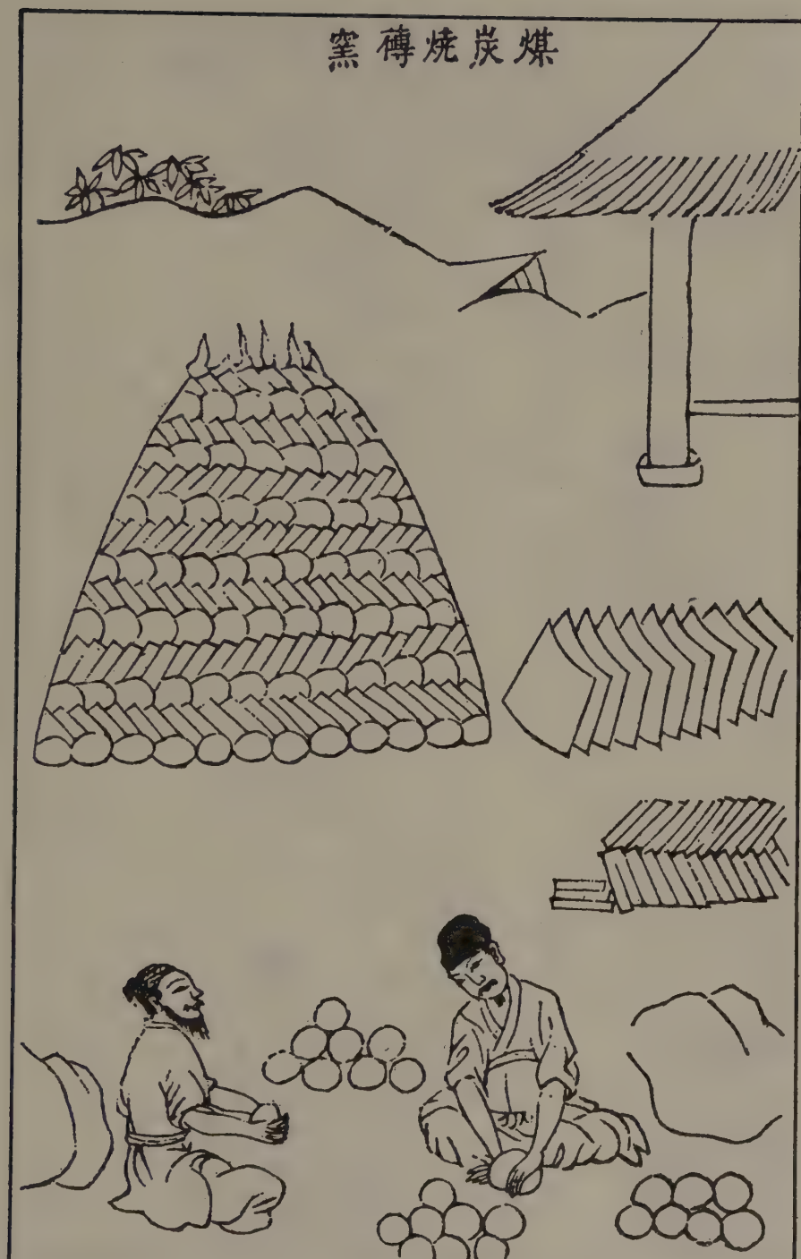
Figure 7-4. Coal-fired brick kiln.
