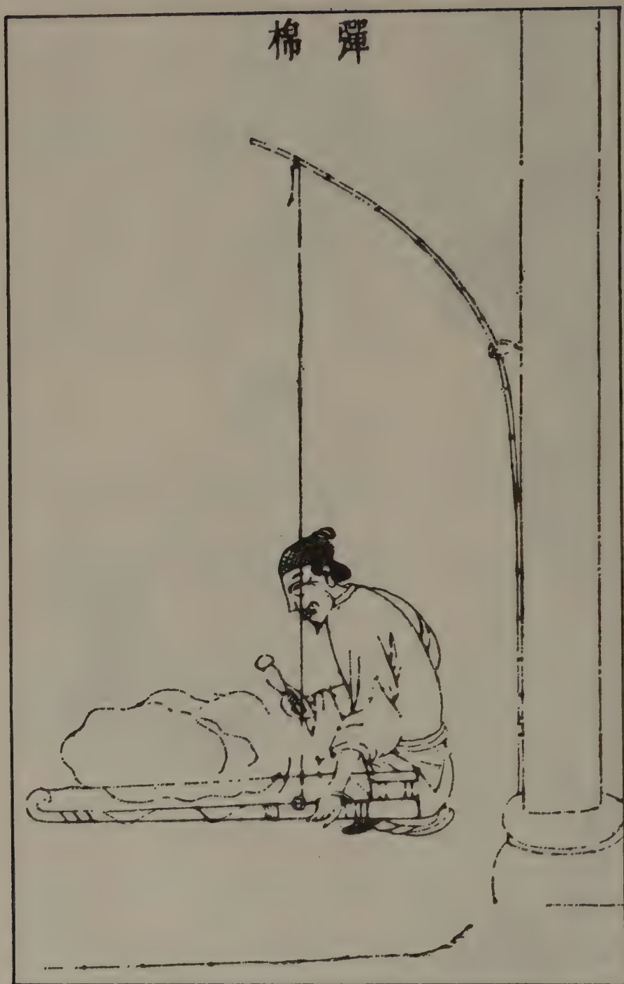
Figure 2-16. Bowing of cotton fibers.
