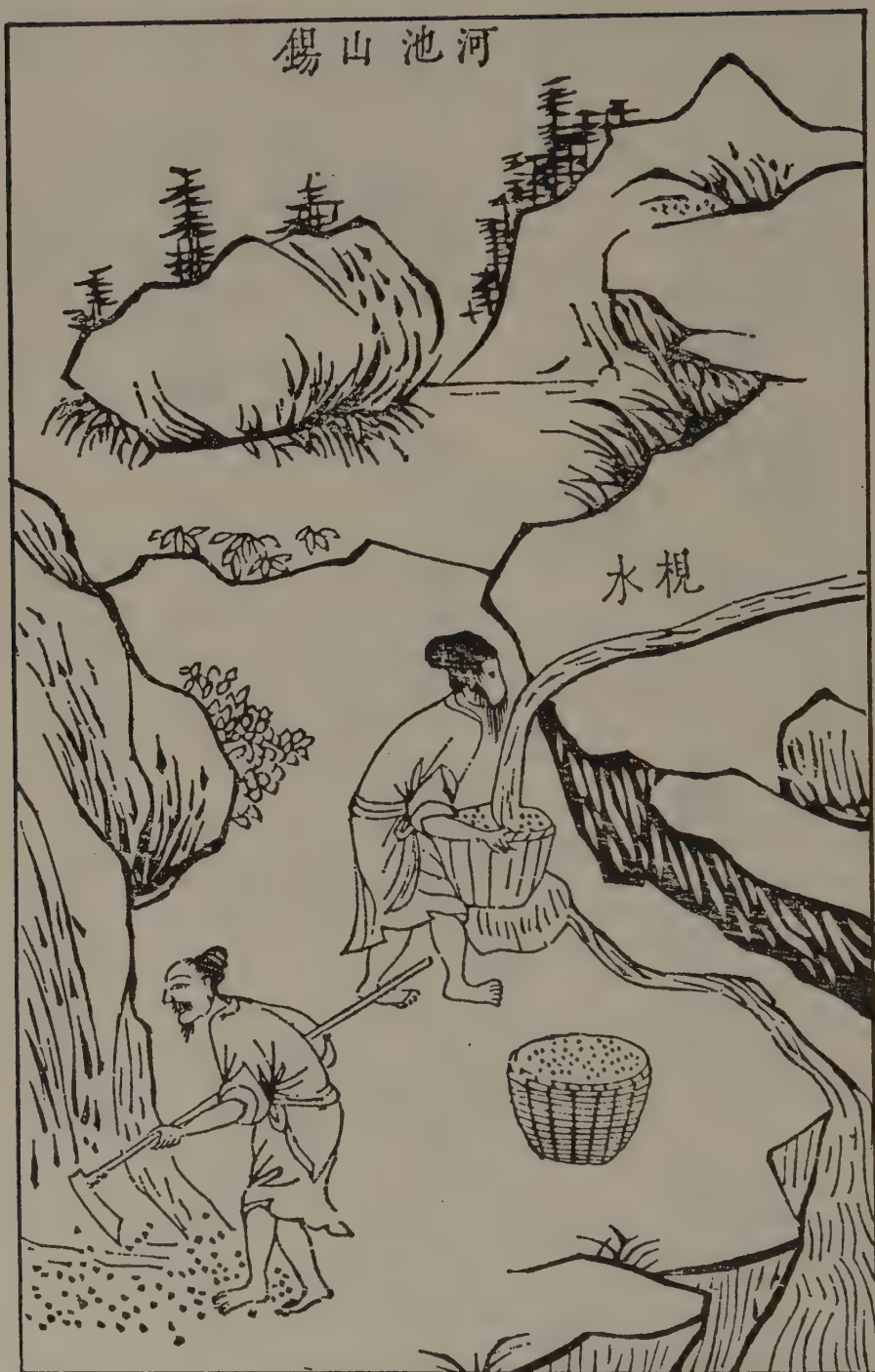
Figure 14-12. Concentrating mountain tin ore by washing, Ho-ch'ih, Kwangsi.
