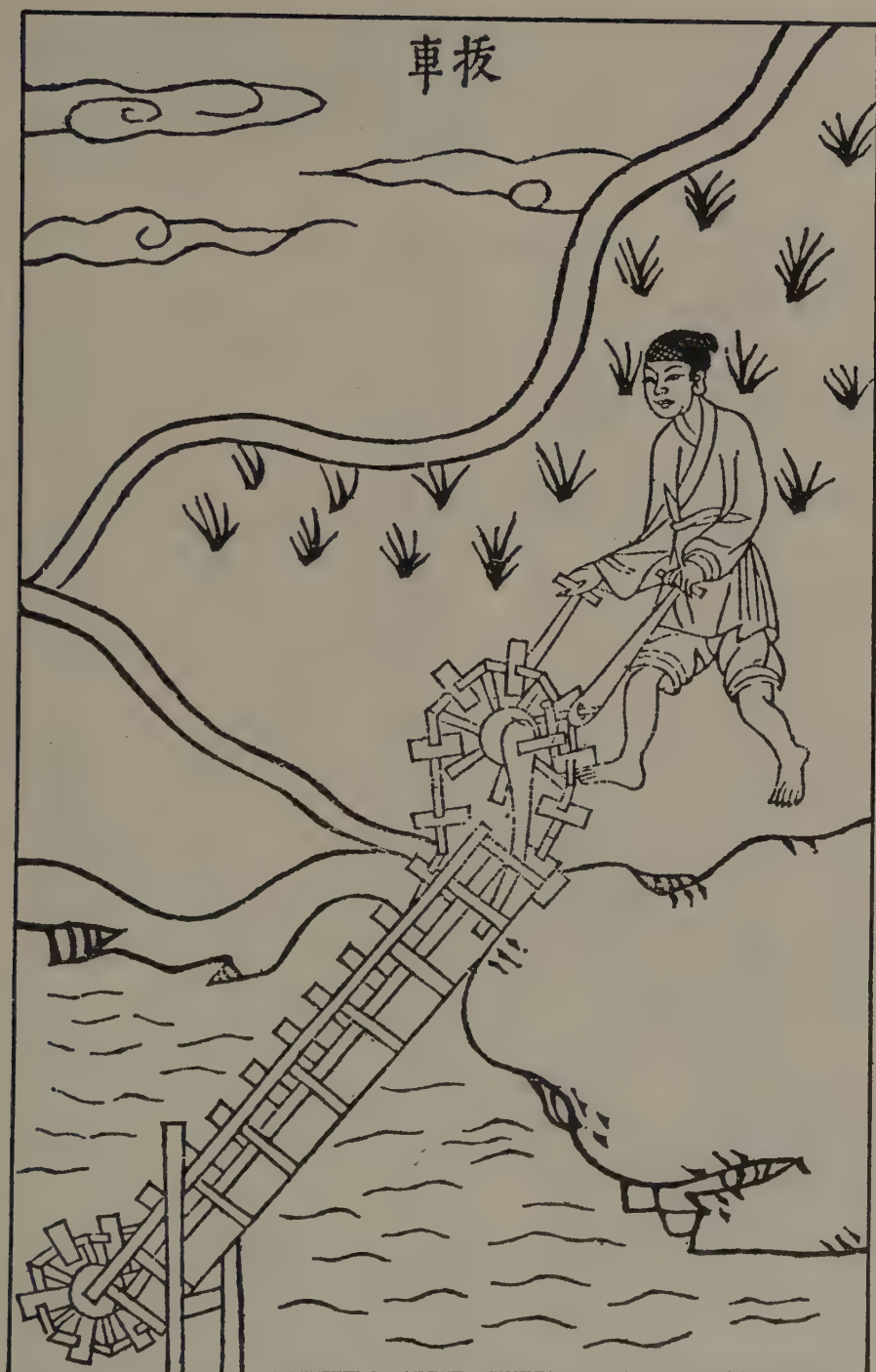
Figure 1-12. Hand cranked wheel.
