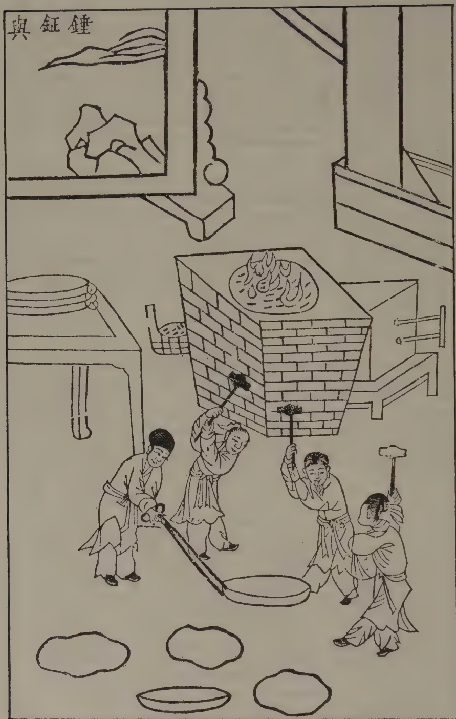
Figure 10-4. First step in making the copper gong and copper drum.
