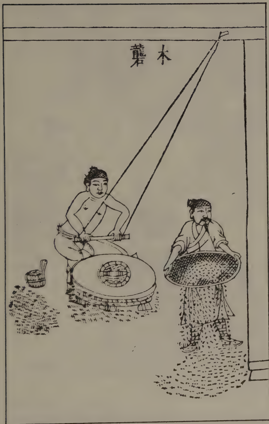
Figure 4-6. A hand-operated wooden hulling mill.
