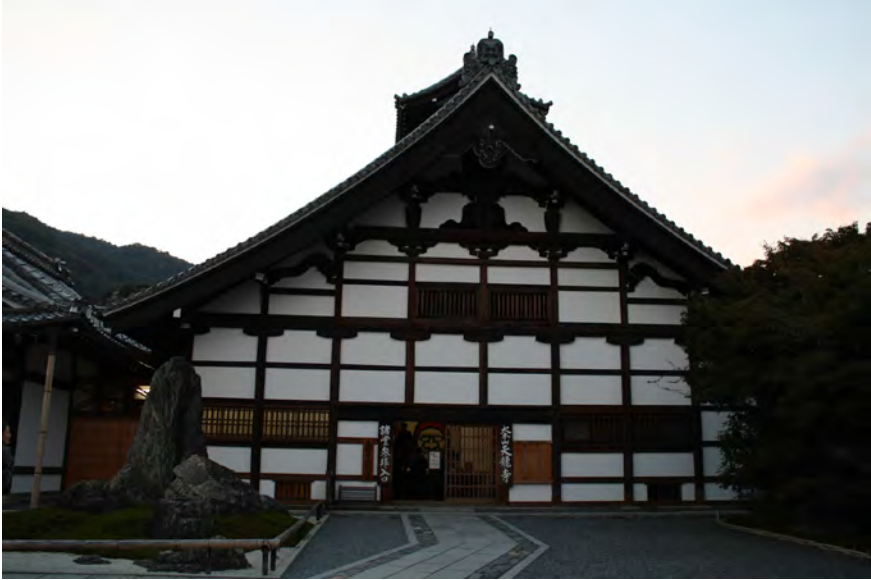
FIGURE 16 Kuri (kitchen) at Tenryūji
