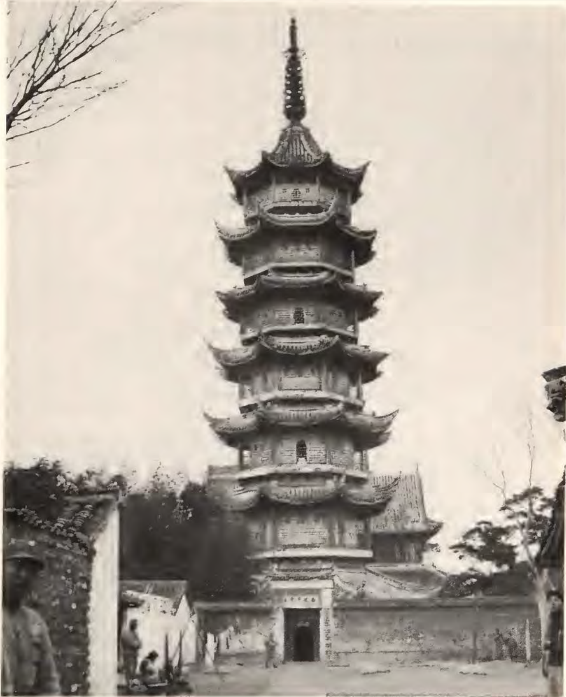
3 The Ch'ung-en Pagoda occupied by troops in the 1930's. Note how the lattice work has been broken in the first-story railing; and how many finials and windbells are missing from the eaves. On the temple building in the rear, the ridge coping has fallen off the whole right end of the roof.
