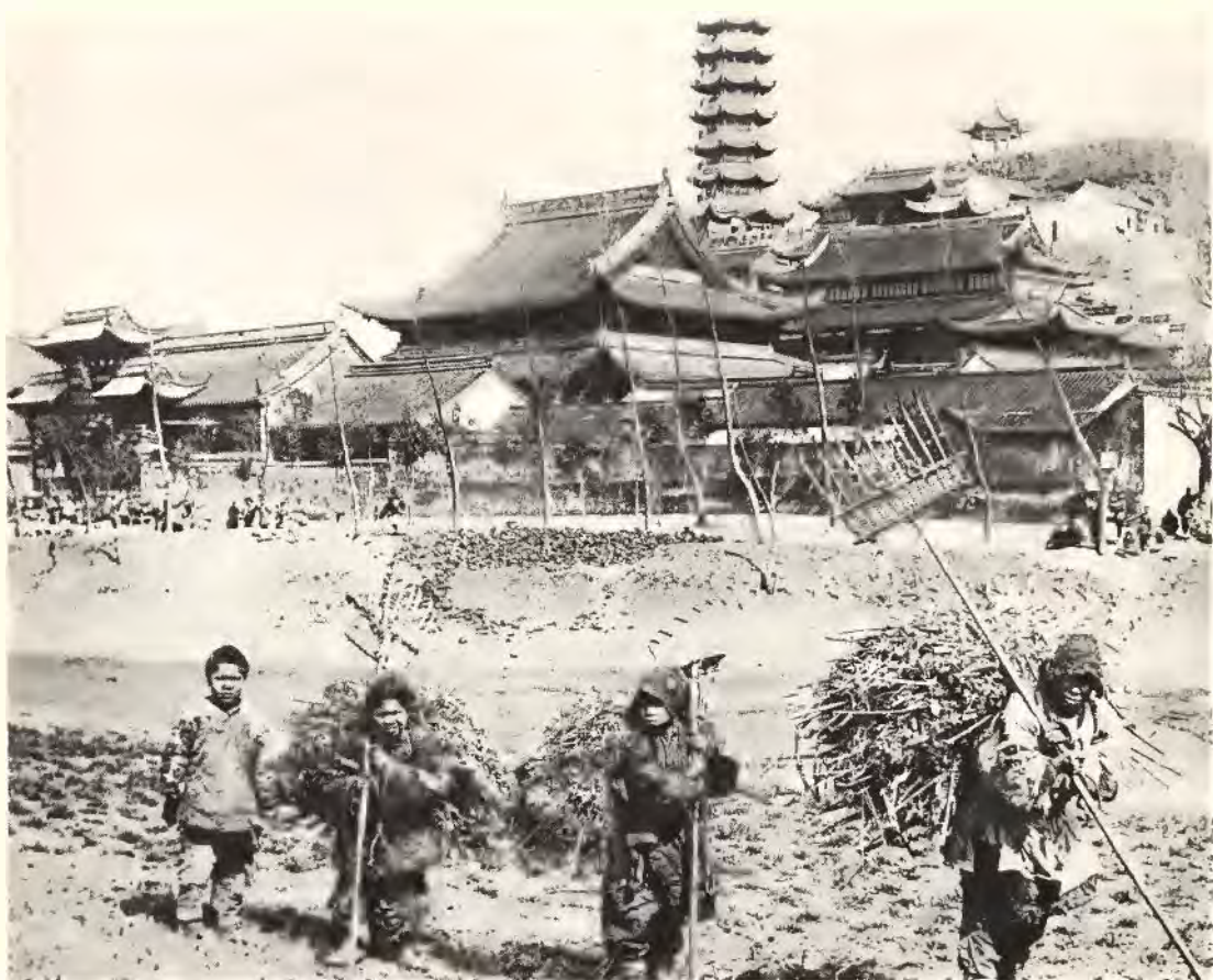
4 Chin Shan. The Kuan-yin Ko stands on the terrace just below the crest of the hill, behind the long, many-windowed library of the Chiang-t'ien Ssu, to which all the other buildings belong. The ragged peasant family in the foreground has been gathering faggots from the monastery's land.
