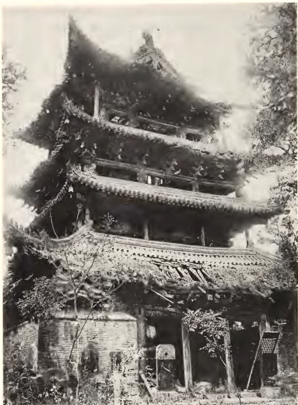
33 The dilapidated drum tower of the Shao-lin Ssu, one of the most famous monasteries of north China, at Sung Shan in 1920.
